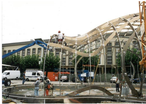
Fig. 8. On-site assembly of the digitally fabricated structural framework, demonstrating the transition from digital model to physical construction guided by CNC-produced components (Hadia, 2007).
